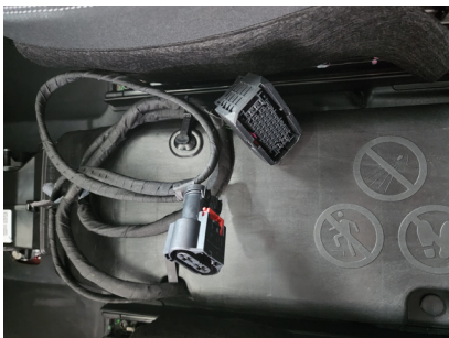
Located under console
